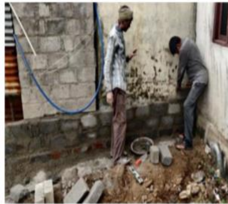
Pilot scale study of Cement Mortar Mix For Wall construction at Children's Park, Mysaiah Nagar, Warangal, Telangana.
